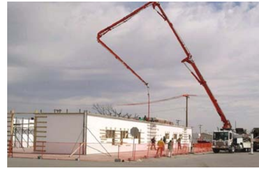
The Greensburg State Bank rebuilds with insulated concrete form construction.
