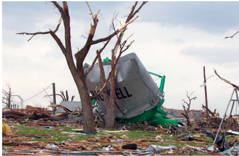
Remains of the Greensburg Big Well Water Tower following a category EF-5 tornado that effectively destroyed the town on May 4, 2007. (Photo by Sean W. Reid.)
